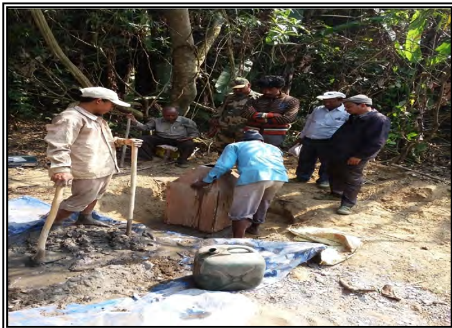
Pillar construction work in International Border in Mizoram- Myanmar Sector
